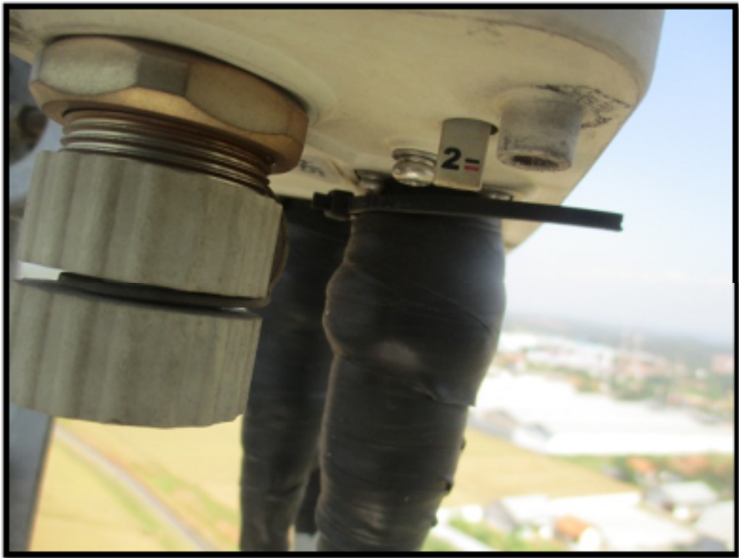
Gambar 2.23 Contoh Pengaturan Electrical Tilt (Edvan Berliansah, 2016)
